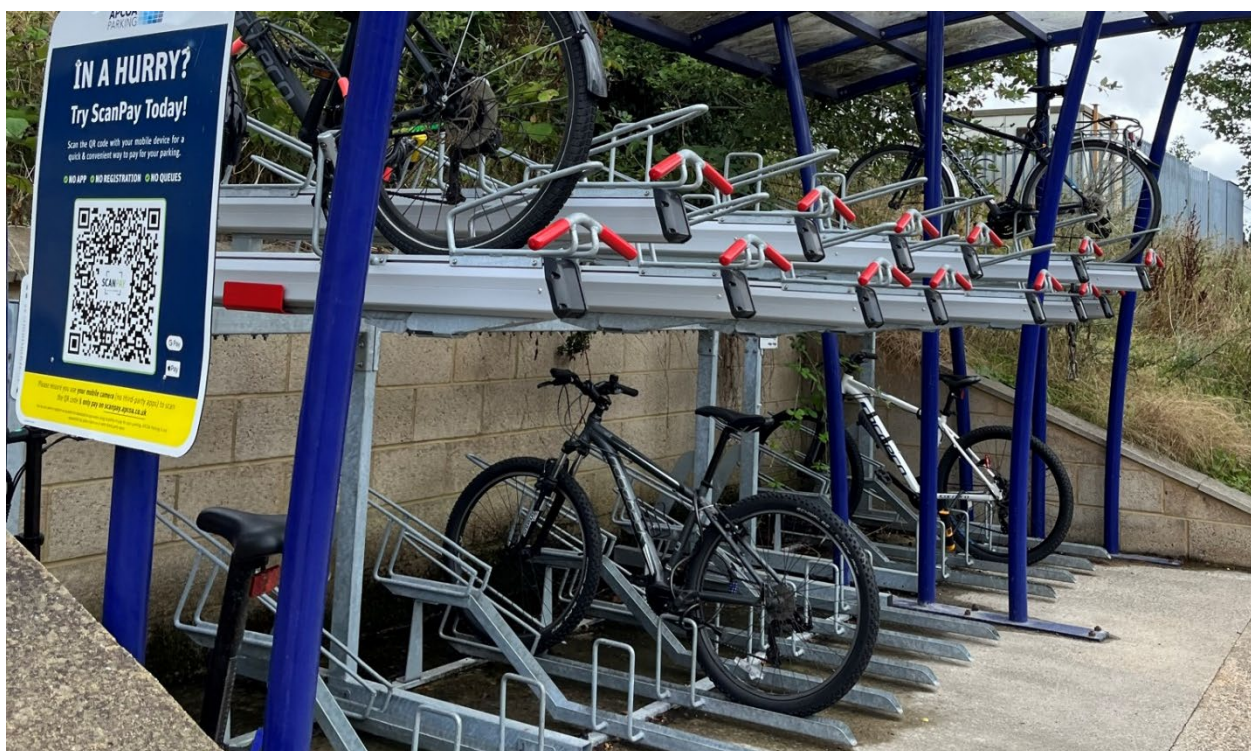
Figure 2-7: Cycle Parking At Baldock Railway Station
